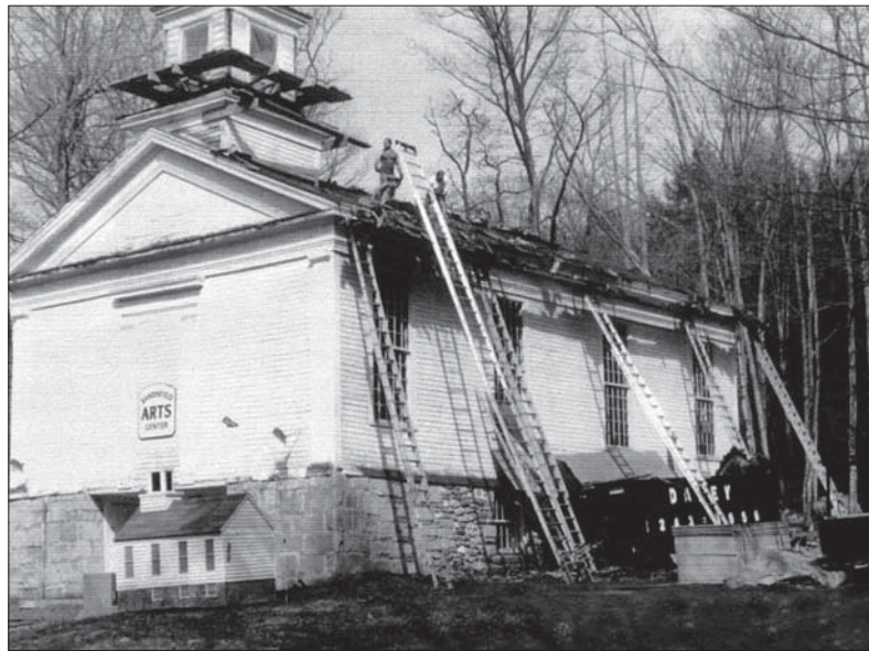
Roof and belfry repairs, May 2000. (Richard Migot)
